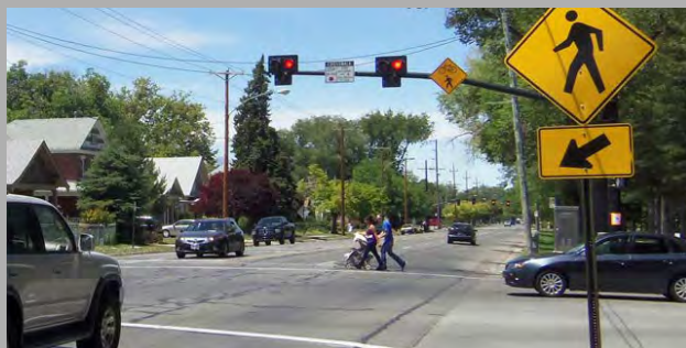
HAWK signals are activated by pedestrians to increase motorists' awareness at crosswalks.
