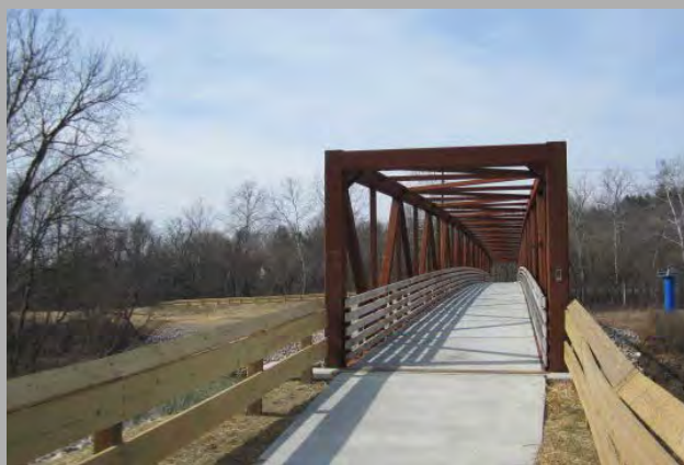
The City of Athens utilized more than $1.2 million in COTF and TAP funding for construction of a regional bikeway connection & pedestrian bridge.
