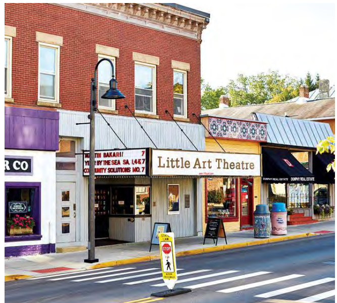
A community's image and brand can be reflected in streetscape design, signage, and public art.
