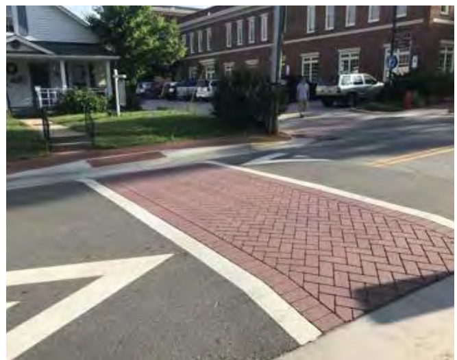
Highlighting crosswalks with patterns and color can help to heighten the level of visibility to motorists.
